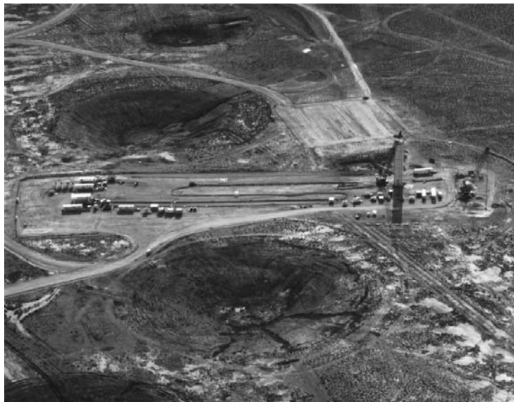
Nevada Test Site. Preparations for an underground test. Final test preparations include running miles of cable downhole which will transmit vital test information to the diagnostic trailers to the left. A rack containing instrumentation to go downhole is assembled in the tower to the right. Subsidence craters from earlier underground tests dot the landscape. (Caption and photo courtesy of National Nuclear Security Administration/Nevada Site Office. (NF-1679) Photo taken 1992 or earlier.)
